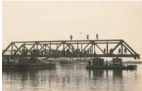
Transfer of Girders by Pontoons Photos: Provided by Fusao Hosono
