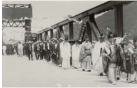
Opening of the Bridge
