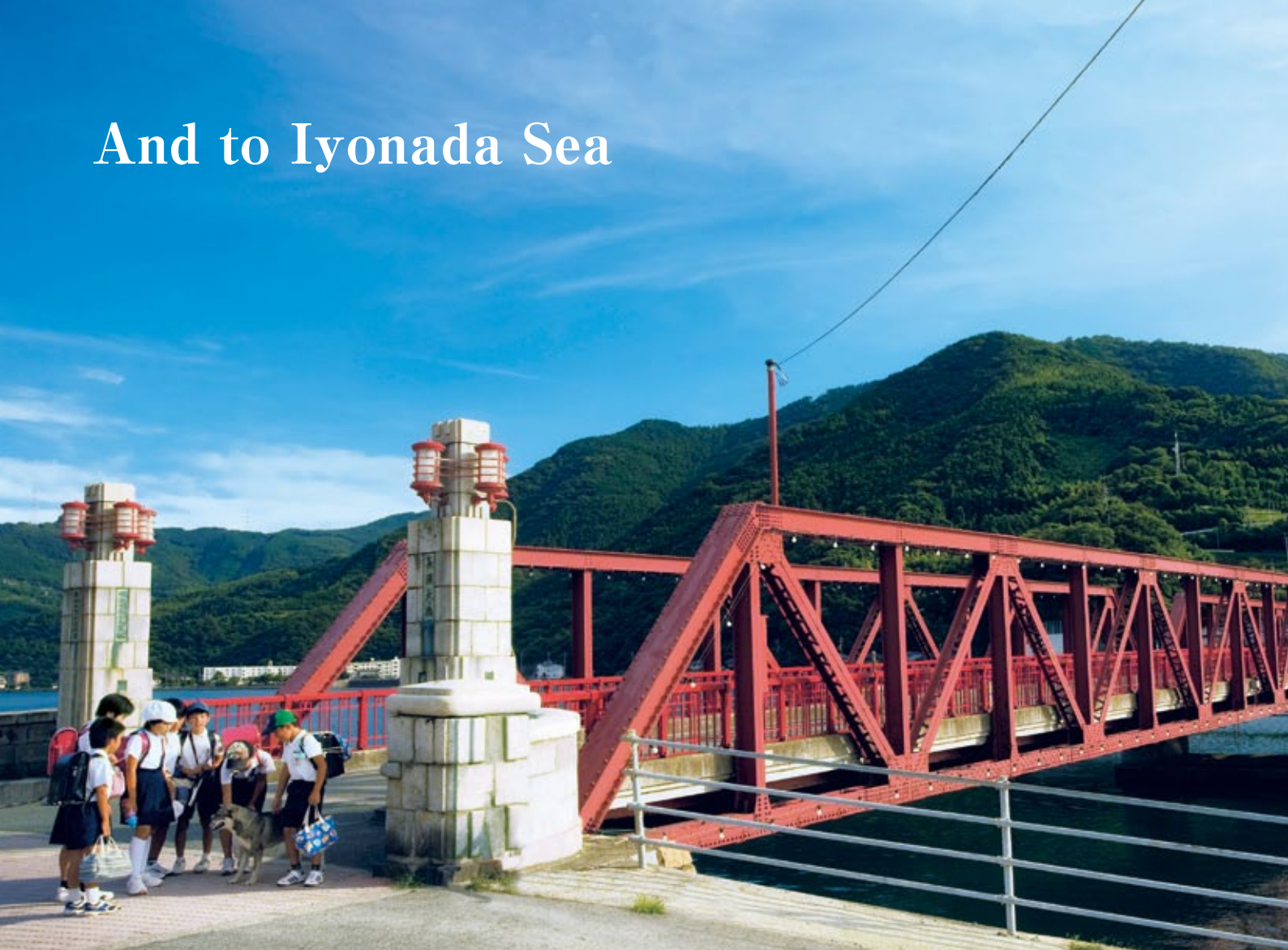
The Nagahama Ohashi Bridge cost 290 thousand yen (in those days) and took two years to construct from 1933
