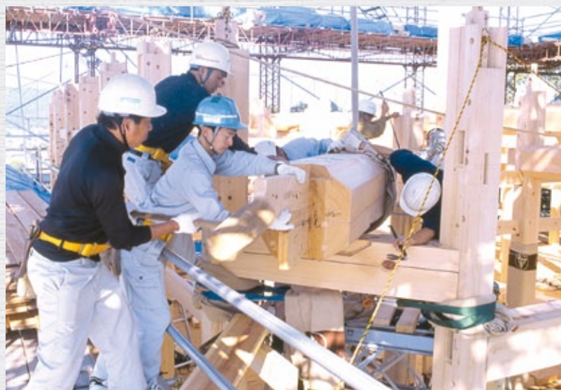
Master craftsmen who were involved in the construction
